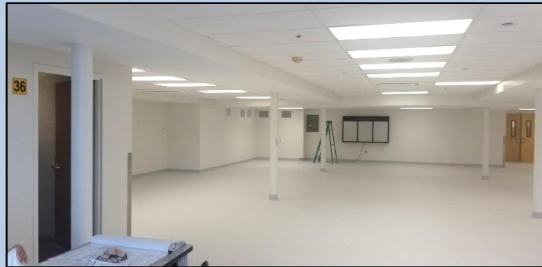
Construction Progress at cafeteria
