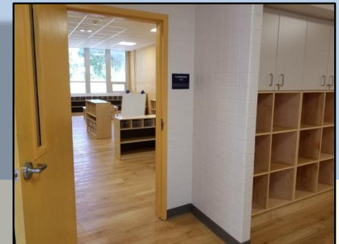
Site Progress Photo
